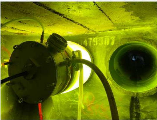
UV Liner in place curing
